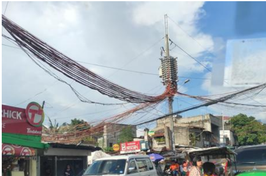
Figure 46. Electric meters on top of posts
